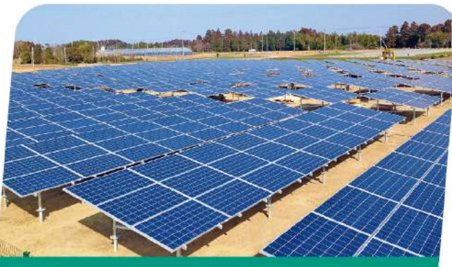
Project size: 2MW Site Location: Japan Finished Time: 2014 Project type: ST1 Steel Ground Mounting
