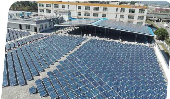
Project size: 8MW Site Location: Barbados Finished Time: 2014 Project type: Concrete Roof Mounting
