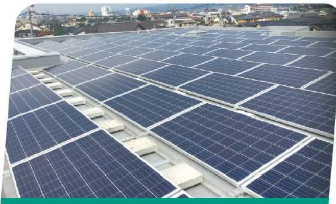
Project size: 8MW Site Location: Japan Finished Time: 2015 Project type: Ballast Mounting
