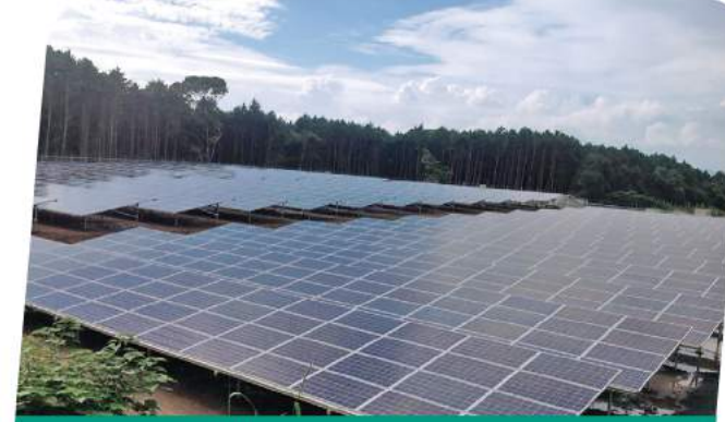
Project size: 7MW Site Location: Japan Finished Time: 2014 Project type: ST3 Aluminum Ground Mounting
