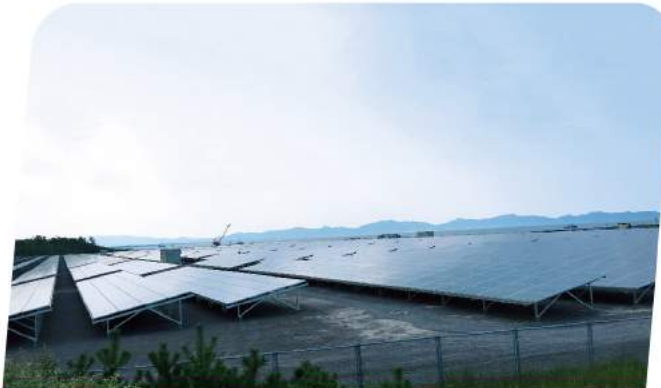
Project size: 30MW Site Location: Netherland Finished Time: 2017 Project type: ST3F Aluminum Ground Mounting
