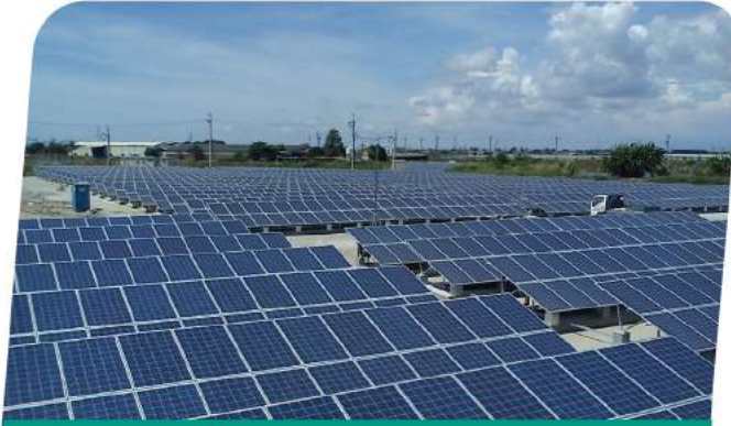
Project size: 10MW Site Location: Japan Finished Time: 2016 Project type: ST3 Aluminum Ground Mounting
