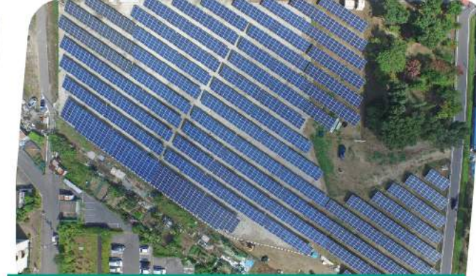
Project size: 1MW Site Location: Japan Finished Time: 2015 Project type: ST1 Steel Ground Mounting
