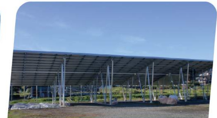
Project size: 350KW Site Location: Japan Finished Time: 2015 Project type: Aluminum Carport
