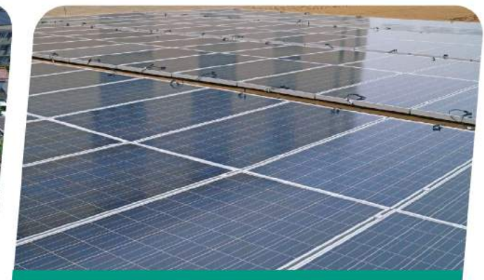
Project size: 3MW Site Location: China Finished Time: 2016 Project type: Trapezoidal Roof Mounting
