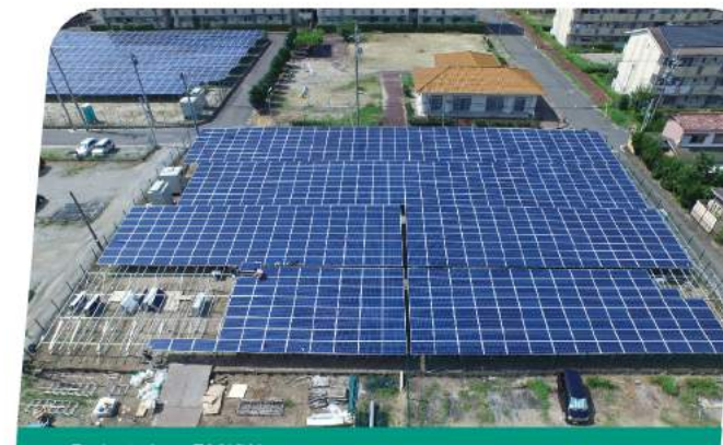
Project size: 700KW Site Location: Japan Finished Time: 2015 Project type: ST1 Steel Ground Mounting
